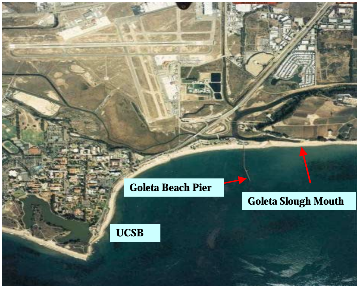
Figure 4.1. Aerial View of the Goleta Slough and Tributaries. Photo Courtesy of Karl Treiberg, Santa Barbara County Flood Control.
