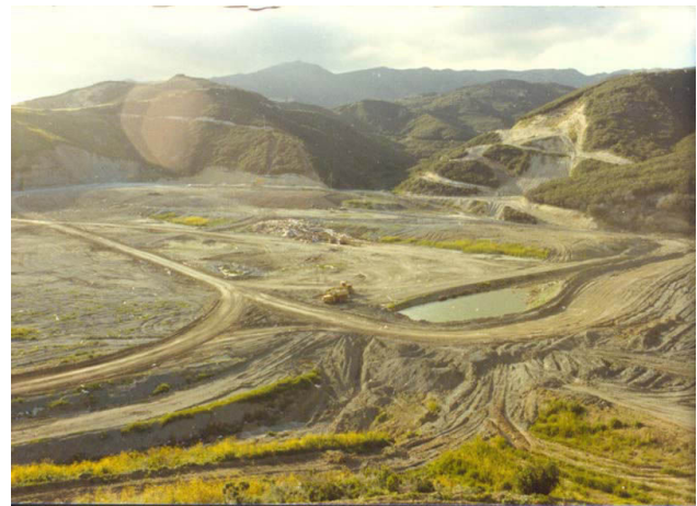
Photograph of Tajiguas Landfill (courtesy of the County of Santa Barbara official website).
